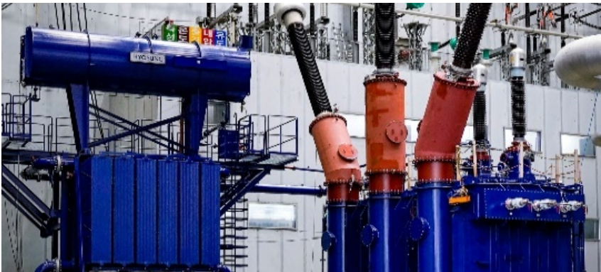
Biodegradable ester oil transformer
