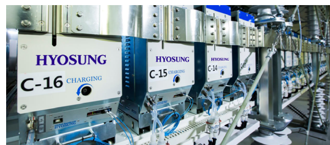
Static Synchronous Compensation (STATCOM) by Hyosung Heavy Industries
