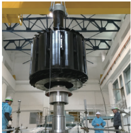
15MW water generator
